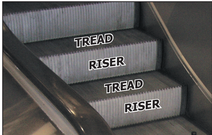
Figure 17. Vertical Face of Escalator is Riser
