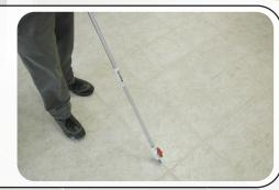
Apply sealer with grout line applicator. Squeegee excess onto grout and wipe up remainder off of non-porous tiles. If a white haze develops on tiles, buff off with white polishing pad and a 175 rpm rotary floor machine.
