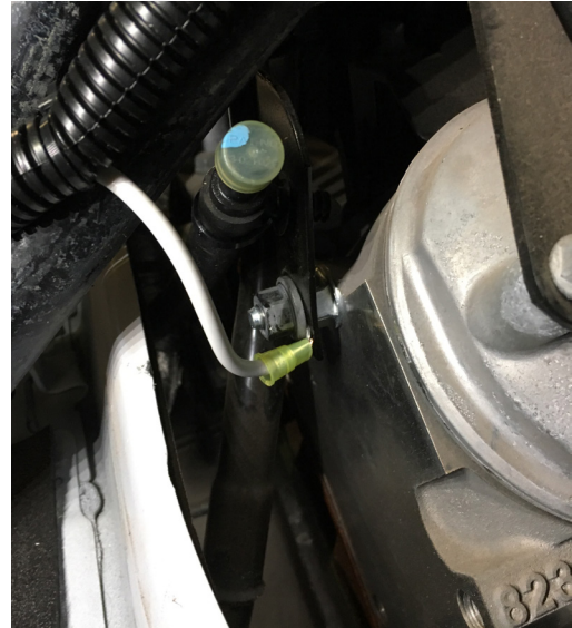
Figure 53. Grounding Location on the Transmission Dip Stick Tube
