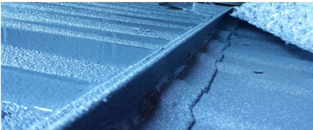
Figure 6. Installed Water Dam with Line-X and the Mat Cut to Length
