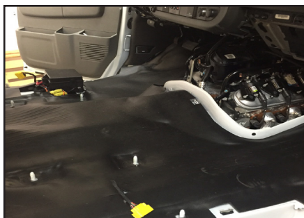
Figure 23. Installed Yaw Sensor cover with front mat laid over it
