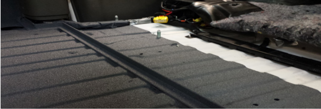
Figure 3. Installed Water Dam with Line-X Coating on the Van's Floor
