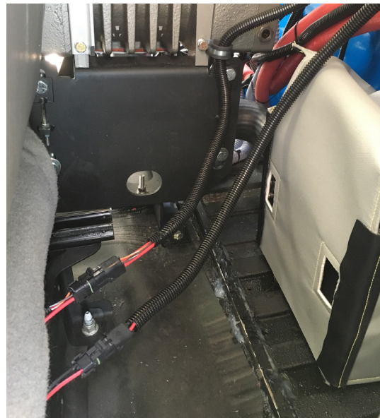
Figure 54. 3 Speed Throttle Cable, Main Power and AWDS Harness (Optional) Off the Floor.
