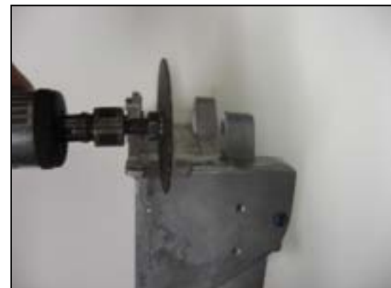
Figure 18. Use Die Grinder to Cut into Bracket
