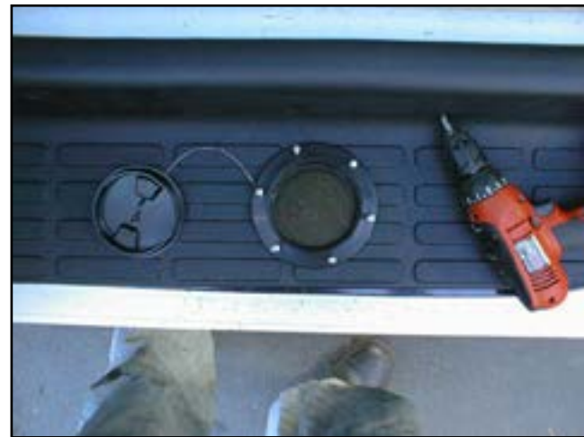
Figure 46. Secure with 6 Self-Tapping Screws
