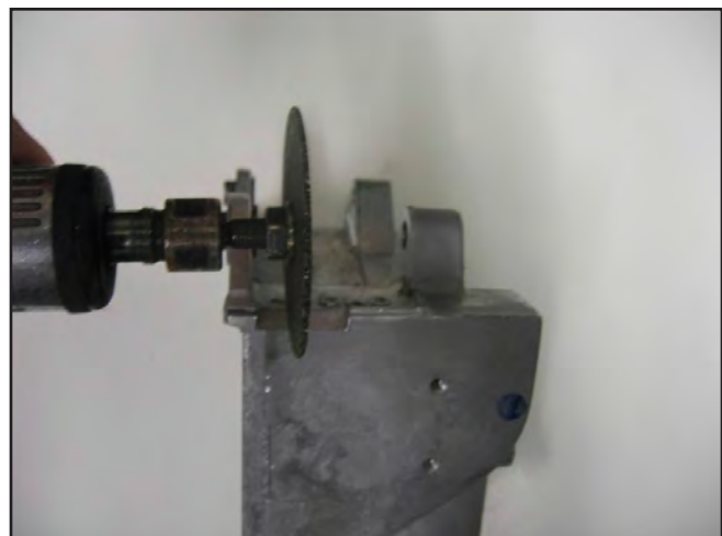
Figure 18. Use Die Grinder to Cut into Bracket
