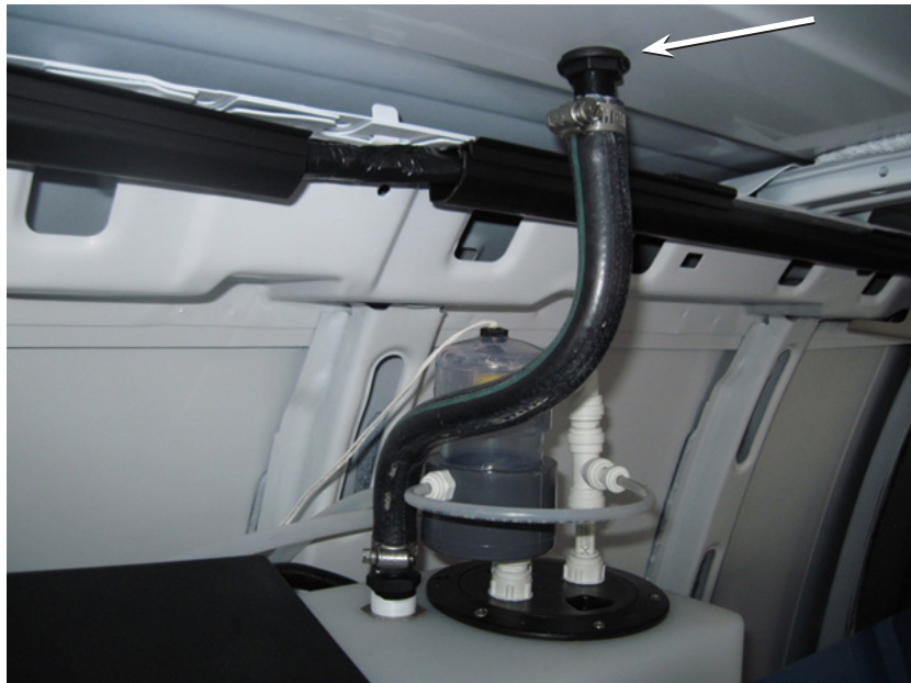
Figure 76. Drill \frac{3}{4} " Hole into Roof of Van
