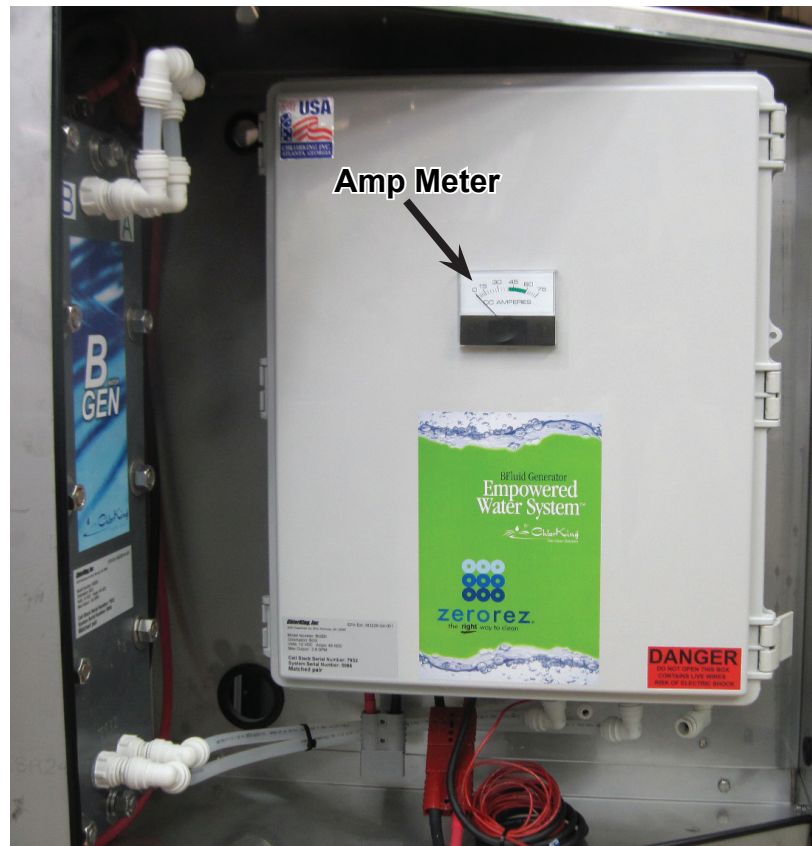
Figure 115. EWS Electric Box and Amp Meter
