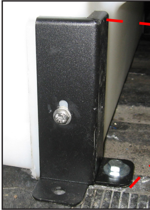
Figure 57. Drill Only 1 Hole for Corner Bracket
