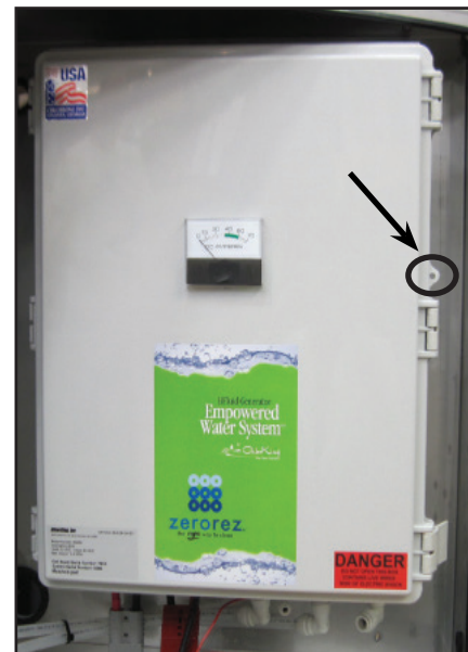
Figure 66. Remove Locking Screw
