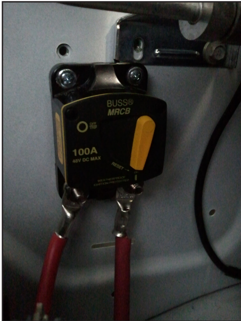
Figure 103. Install Circuit Breaker (Shown without Red Boots)
