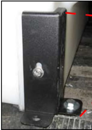
Figure 23. Drill Only 1 Hole for Corner Bracket
