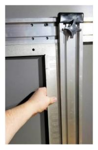
Square the vertical member and secure the vertical member to the sliding plate in the lower rail.
