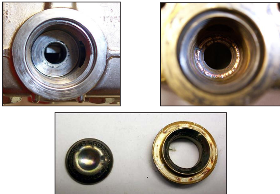
Figure 5-2. Inspect Manifold and Old Valves
