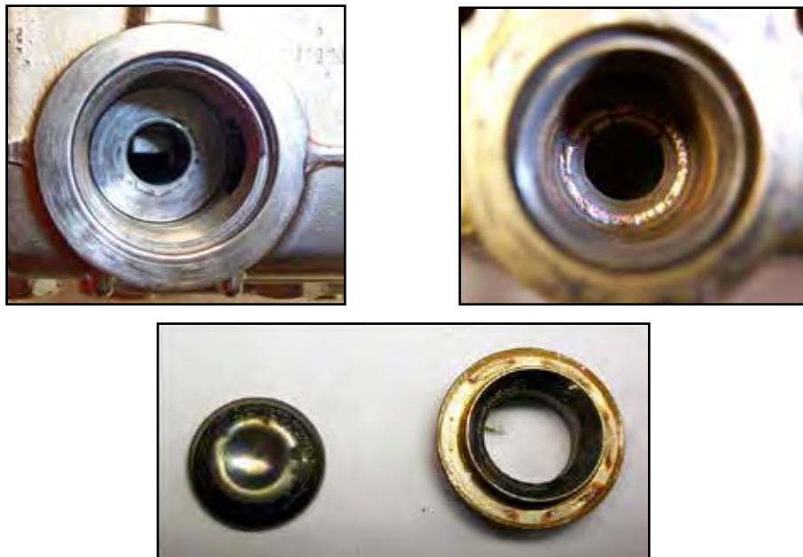
Figure 4-2. Inspect Manifold and Old Valves
