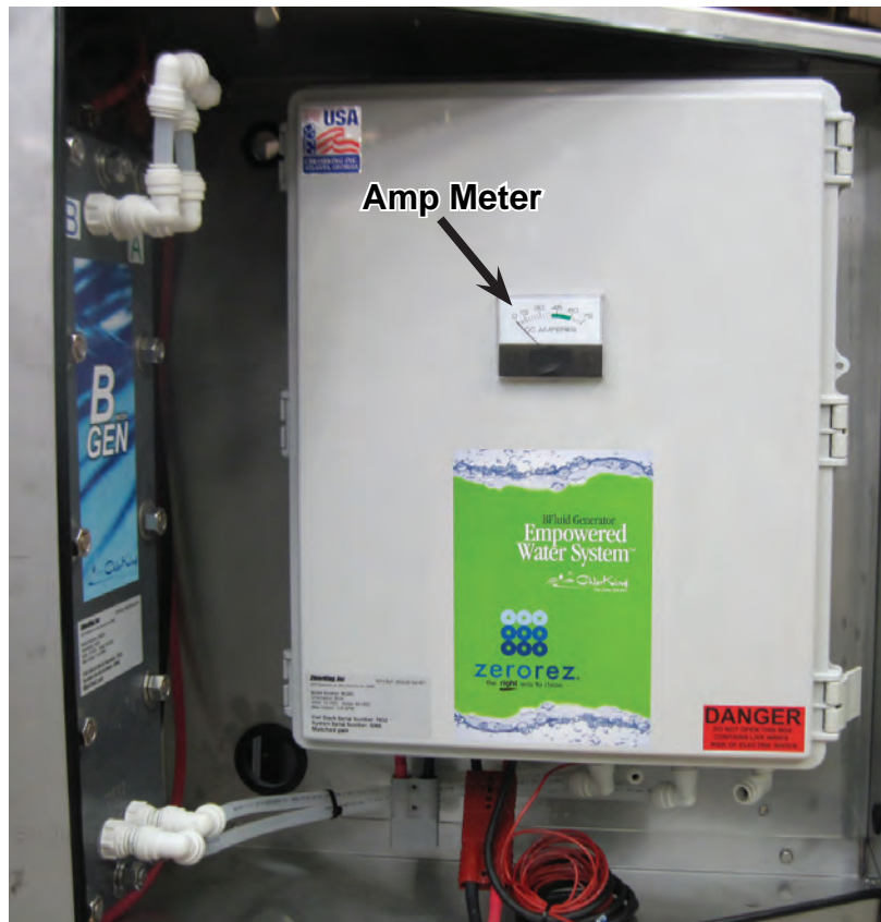
Figure 2-3. EWS Electric Box and Amp Meter
