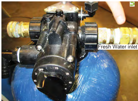
Figure 2-5. Connect Fresh Water Hose to Fresh Water Inlet
