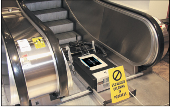
Figure 3. TreadMaster Shown in Preferred Placement, at Bottom of Escalator
