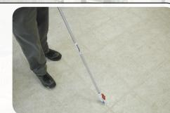
3 Apply sealer with grout line applicator. Squeegee excess onto grout and wipe up remainder off of non-porous tiles. If a white haze develops on tiles, buff off with white polishing pad and a 175 rpm rotary floor machine.
