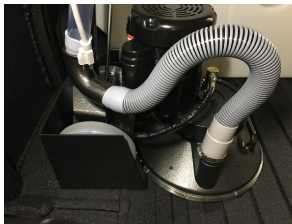
Figure 6-9. Properly stored unit in the storage bracket.
